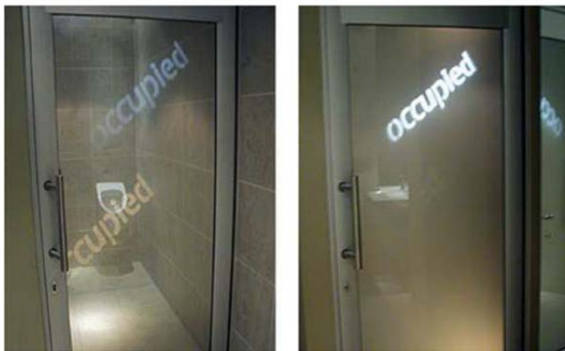
Image 1: Electrochromic glass (Science of Architecture, 2008).
